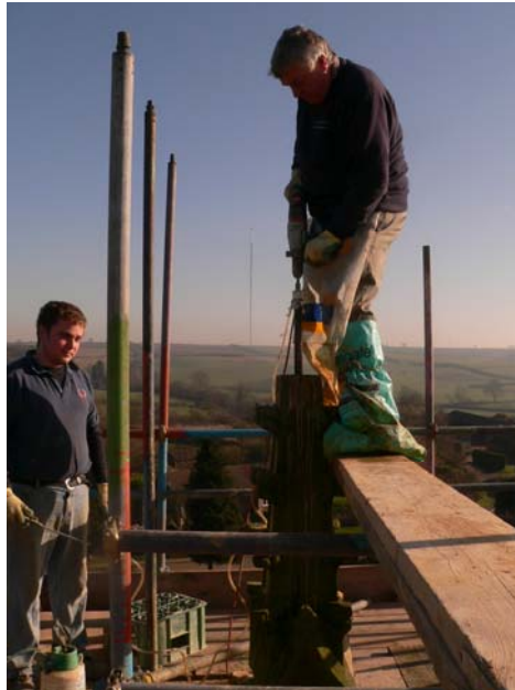
Mick drilling out the core from a pinnacle in order to remove it.
