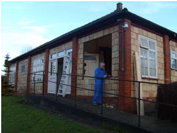
Renovations to the Parish Hall by Jim Fairburn underway (Photo Eric Payne)
