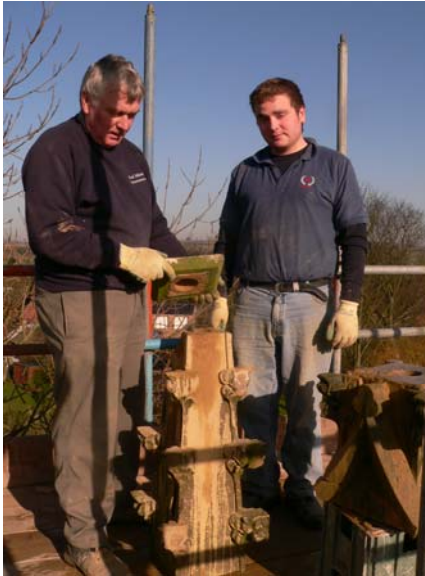
Mick and Ben with part of a pinnacle already in pieces and badly eroded
