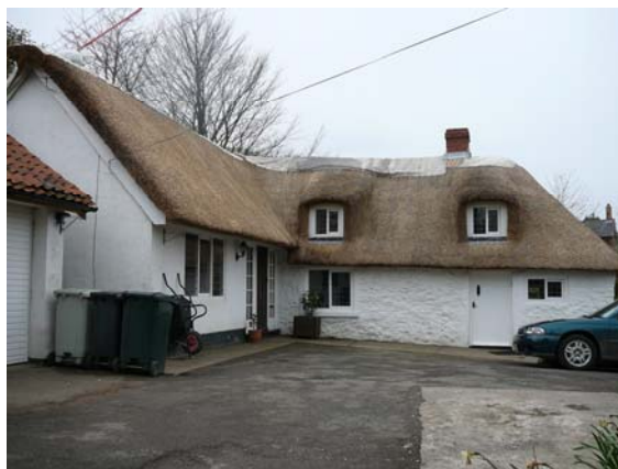
Front of The Thatch almost complete Picture: Liz Noblet
