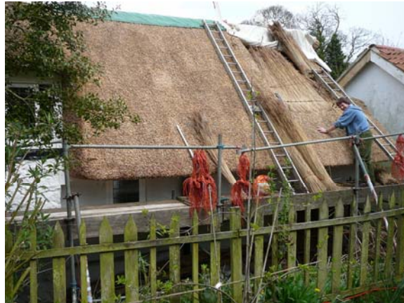
Andrew Bramley hard at work on the back of The Thatch Picture: Liz Noblet
