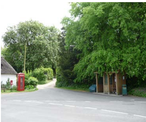
Bus shelter and seat to be renovated
