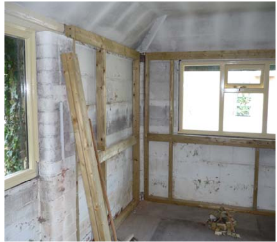
Above is the kitchen stripped and with battens fixed ready for the boards. Now you see the window, now it has gone (below)
