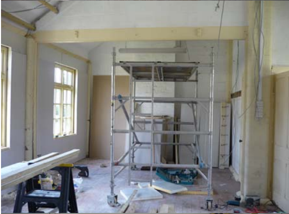
Stages in the refurbishment of the main hall (left). First the walls are stripped, then (middle) the boarding is in place and (bottom) the roof is dealt with.
