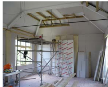
Scaffolding in place as the Hall is renovated.
