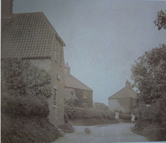
Barkwith Road with Cobbler's Cottage on the left
