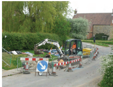
Final (??) repairs to Station Road in full swing
