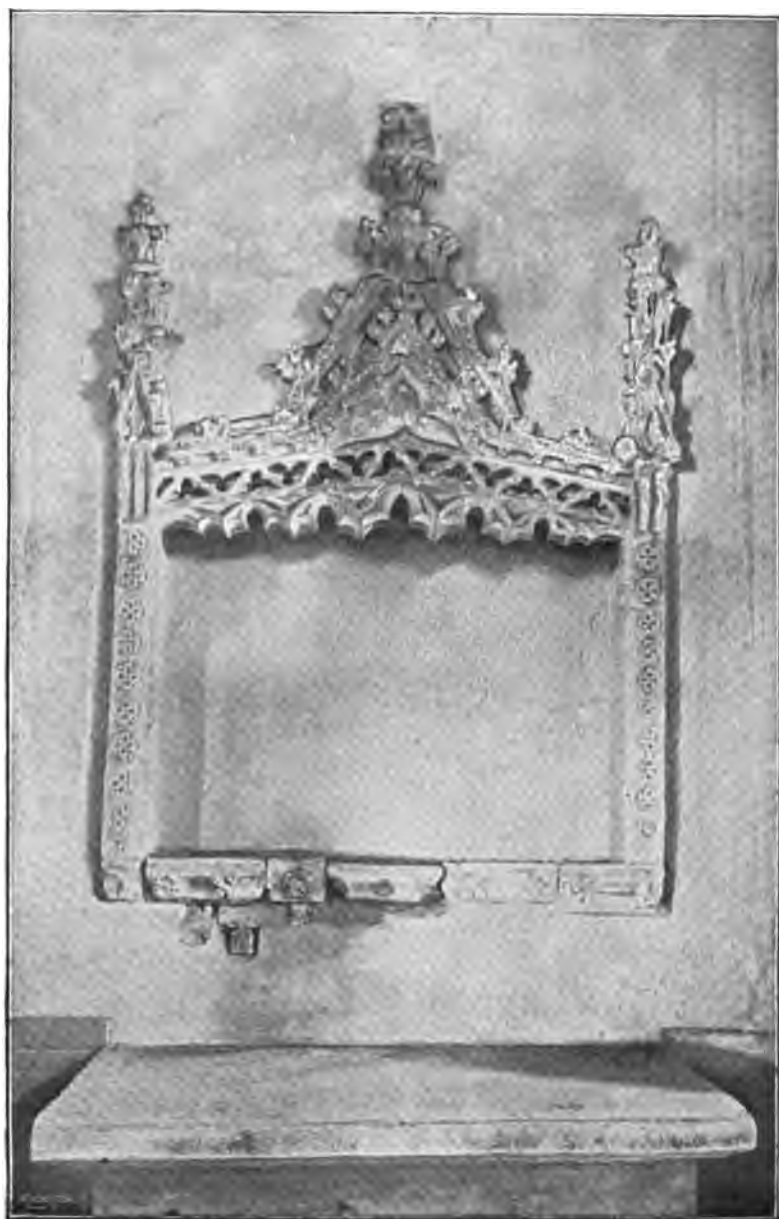
CANOPY AT THEDDLETHORPE ALL SAINT'S CHURCH.
