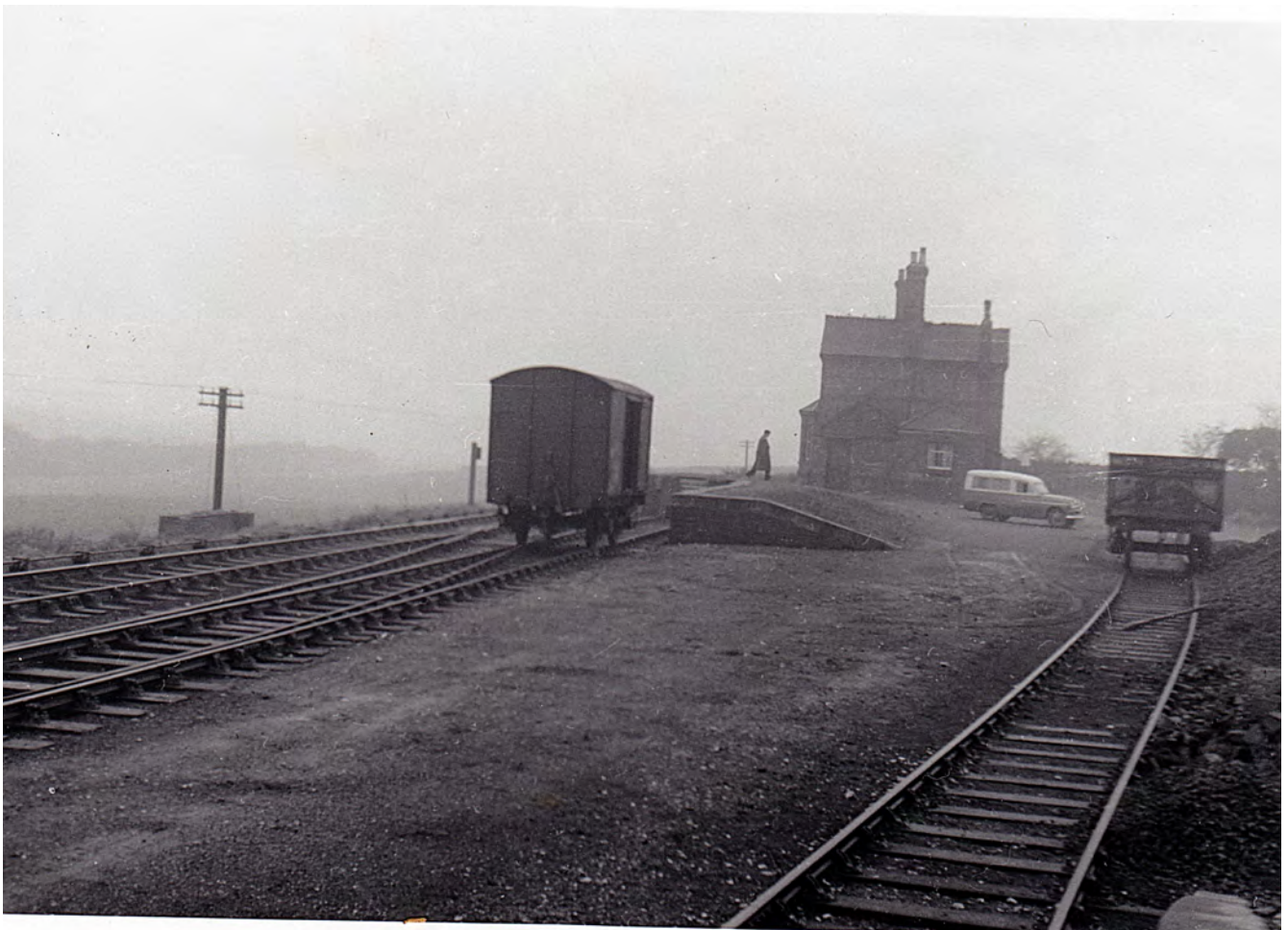
A DESOLATE VIEW IN JANUARY 1958 OF THE GOODS SIDINGS A YEAR AFTER CLOSURE TO FREIGHT. A FORLORN CATTLE WAGON REMAINS NEXT TO THE CATTLE RAMP AND AN EMPTY COAL WAGON NEXT TO THE COAL STAITHES.
