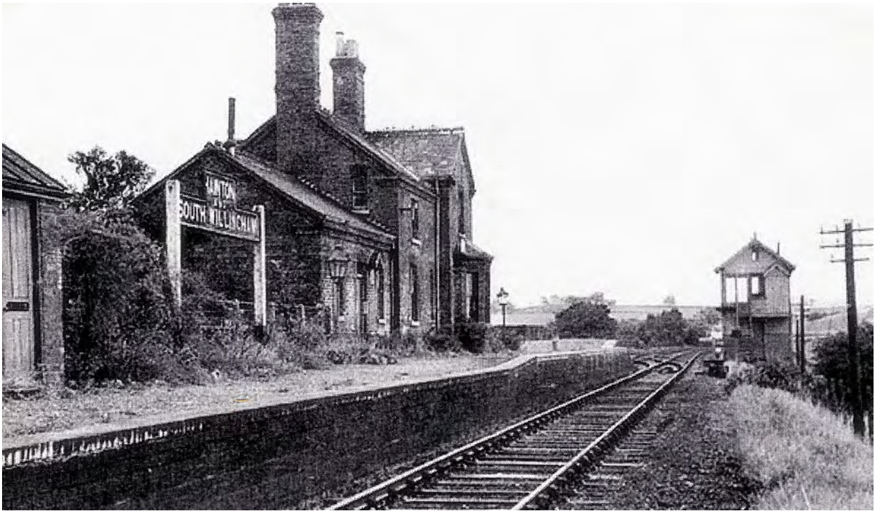
A SAD VIEW OF THE STATION CIRCA 1957, 6 YEARS AFTER THE LAST PASSENGER SERVICE AND A YEAR AFTER THE LAST GOODS TRAIN
