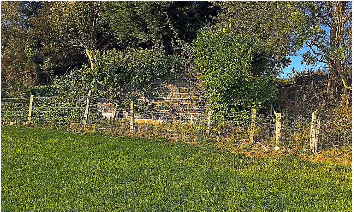
ORIGINAL BRICK BASE OF GNR SIGNAL BOX (PHOTO TAKEN FROM FIELD OPPOSITE STATION) OCTOBER 2018 (PHOTO N.SPENCER)
