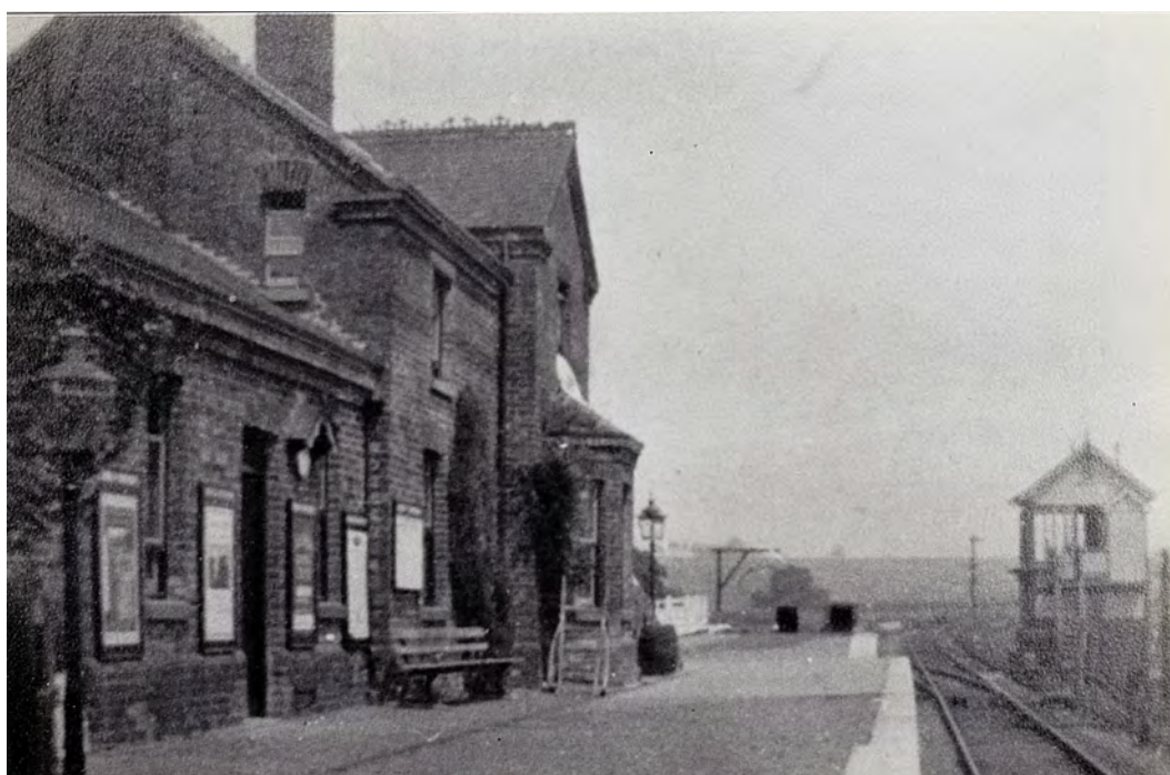
PLATFORM VIEW LOOKING TOWARDS STATION ROAD RAILWAY BRIDGE. THE SIGNAL BOX IS ON THE RIGHT, LOADING GAUGE IN THE GOODS SIDINGS, PORTERS BARROW BY THE SEAT. THE CLOCK IS ON THE WALL WITH A LITTLE ROOF TO PROTECT IT FROM THE ELEMENTS. THE SECTION INCLUDING THE BAY WINDOW WAS THE STATION MASTERS HOUSE.
