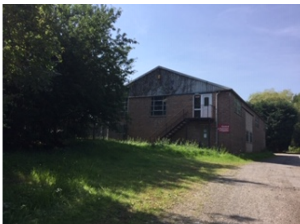
The Sack Building - now Harrison Engineering (Photo: Nigel Spencer)
